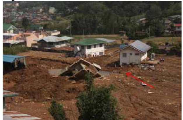
Photo 5.2.2 Photo of damaged area in Barangay Puguis
