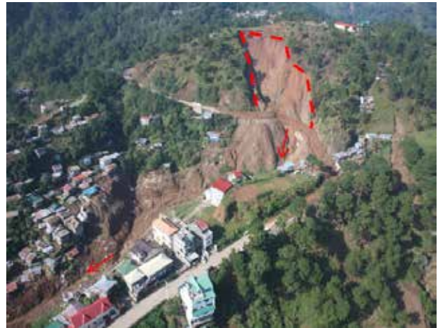
Photo 5.2.1 Aerial photos of damaged area in Barangay Puguis
