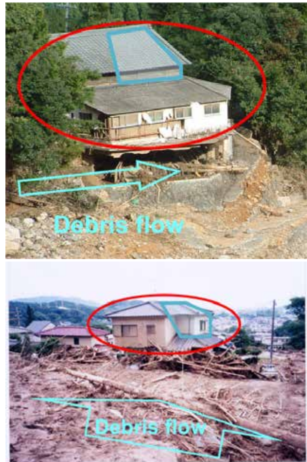
Fig. 2.8.1 No damage to a room on the second floor
