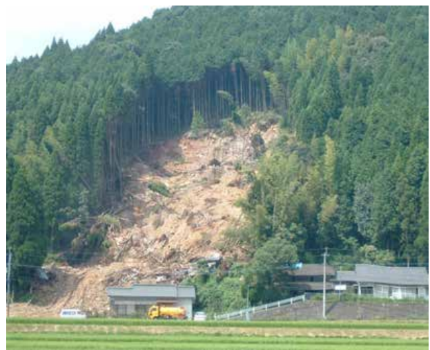
Photo 3.1.3 Slope failure (2006, Hishikari town, Kagoshima pref.)
